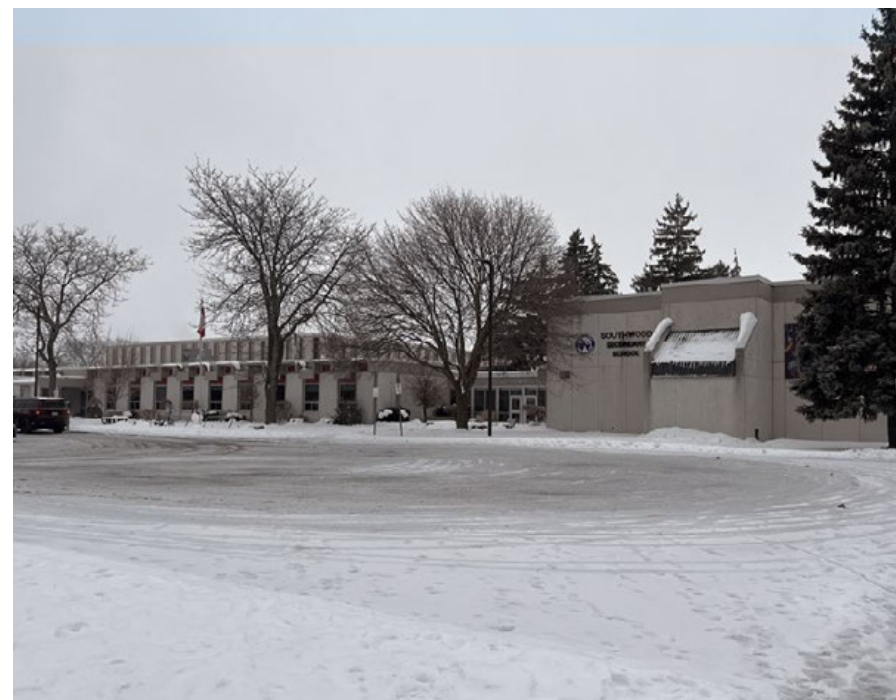
Fig. 1.15 Photo demonstrating experience of arriving at Southwood Secondary School
