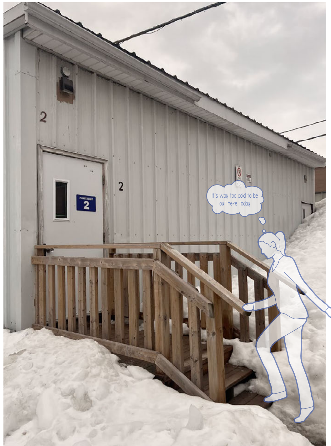
Fig. 1.23 Entrance of a portable classroom on site
