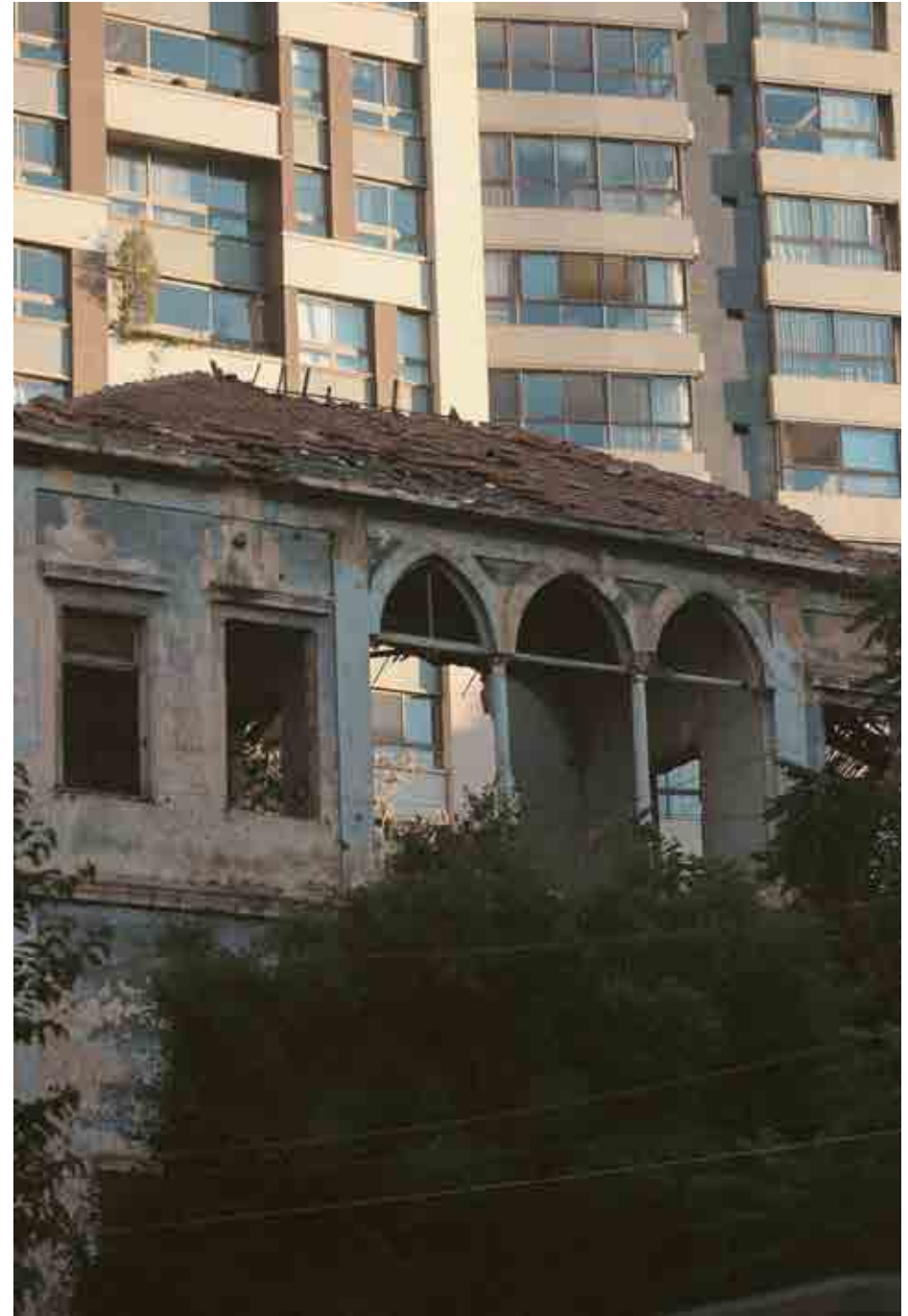
67. Beirut in 2025, Ottoman era abandoned building.
